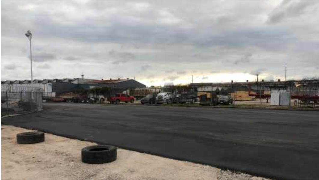
Asphalt paving of parking lot.
