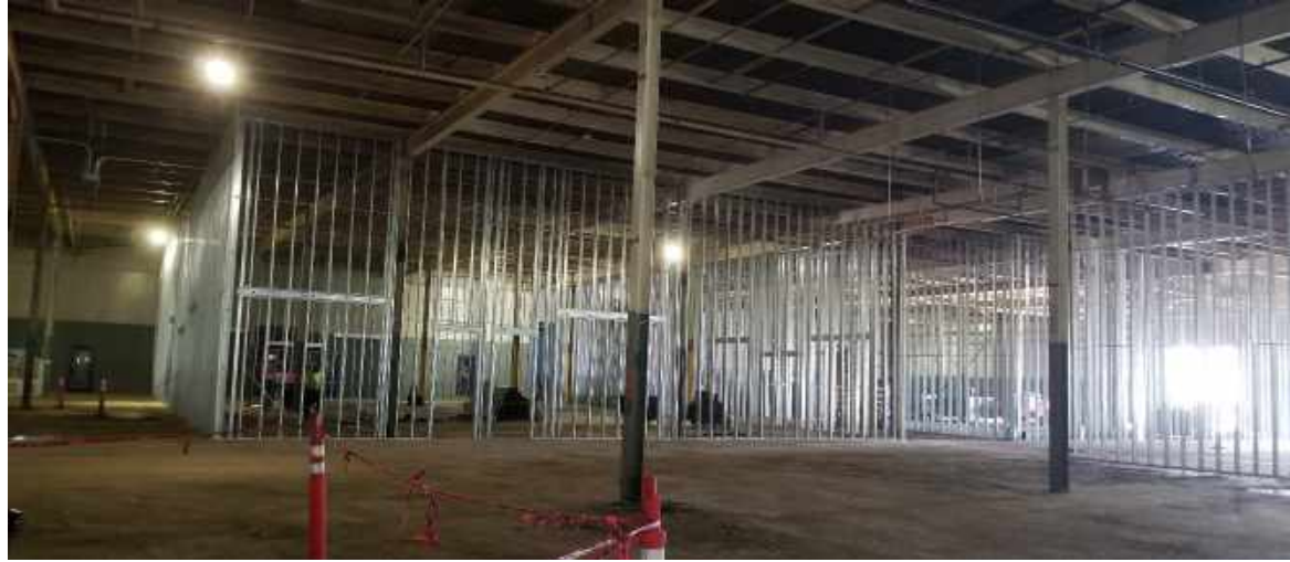
Floor-to-roof metal studs near southwest corner of building.
