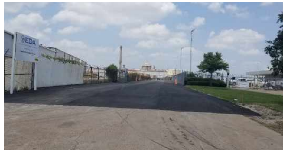
Asphalt paving of west entrance driveway.
