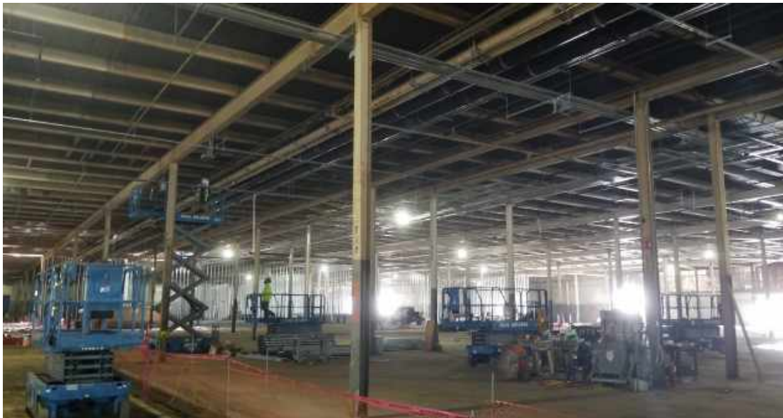
Electrical conduit installation in central area of building.
