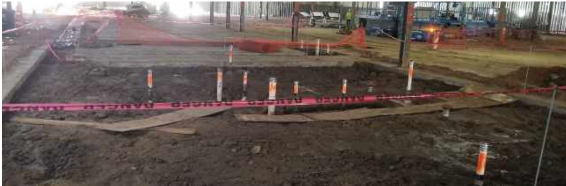
Restroom plumbing stub outs ready for concrete.
