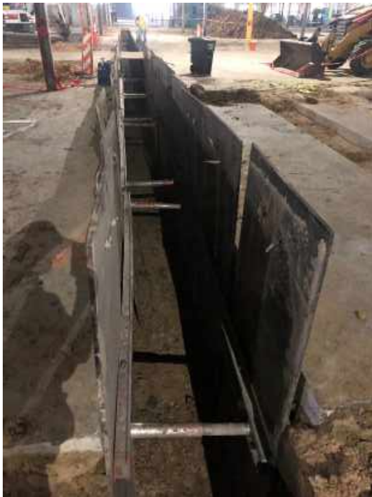
Open trenches for sewer distribution.
