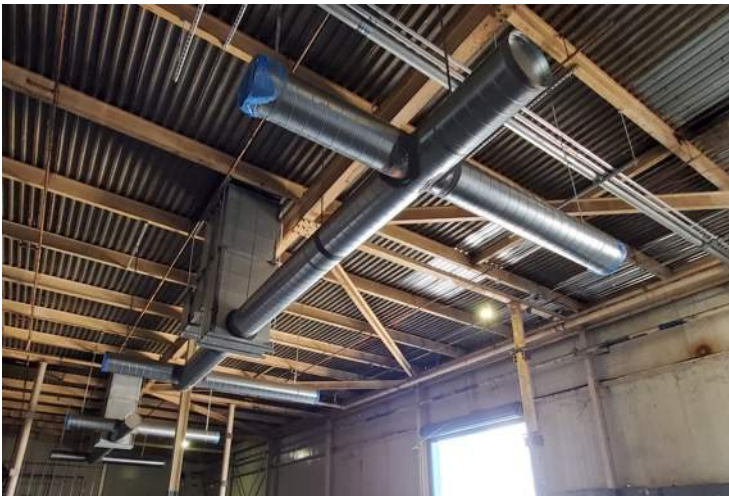
New HVAC distribution ductwork
