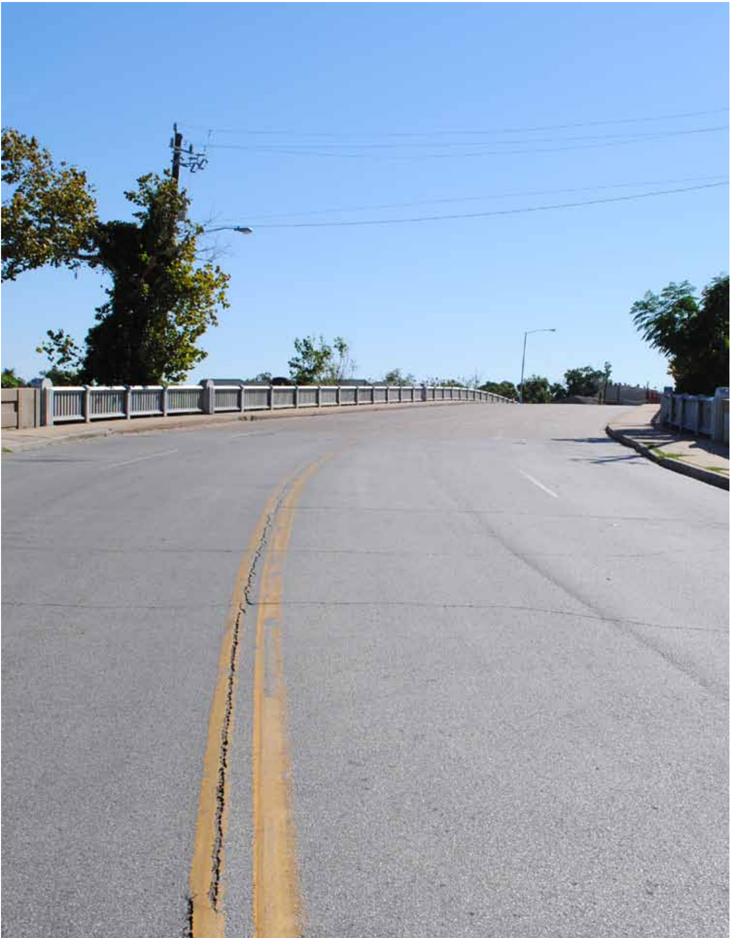
Jensen Street Bridge over Buffalo Bayou
