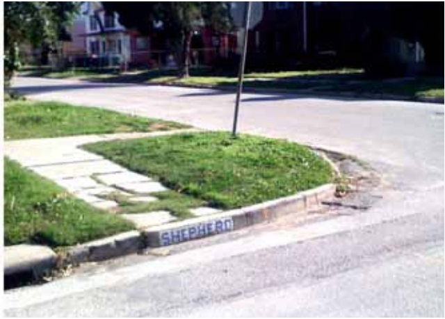
Figure 4.15 This historic tilework has survived the change of the street name. While this form of pedestrian signage is often removed or damaged during the addition of ADA compliant ramps, saving or replacing the tile work can provide an interesting historic brand for the area that also improves pedestrian experience.
