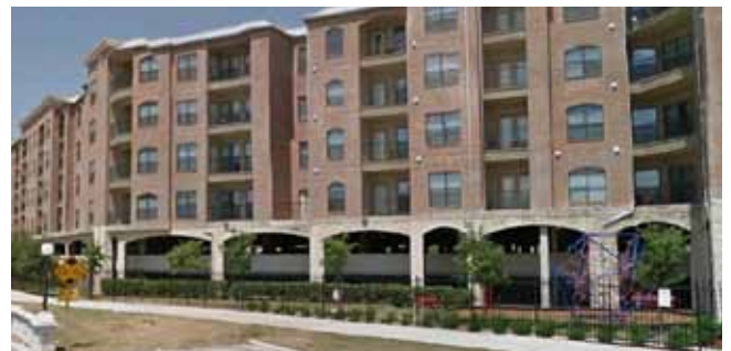
Garage Parking Structure (Canal Place)
